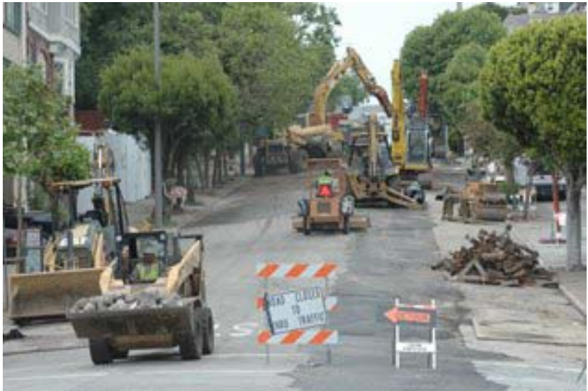
Construction blocks traffic on Pacific between Pierce and Scott
